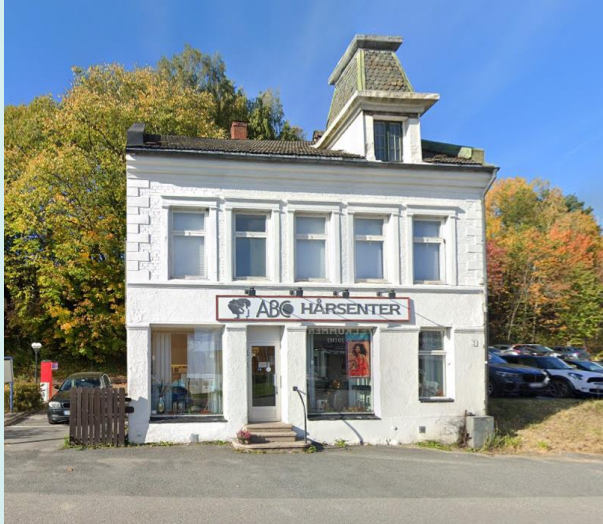
Figur 1 Askveien 3, google street view.
