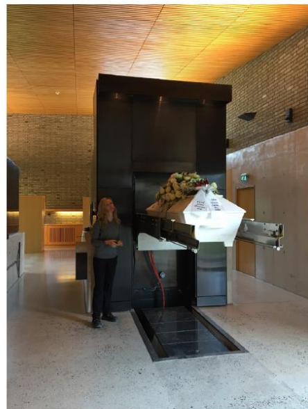
Vestfold Krematorium, ovnsrom
